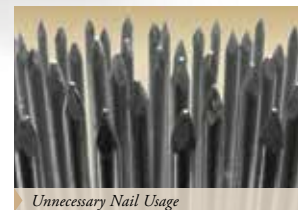
Unnecessary Nail Usage
